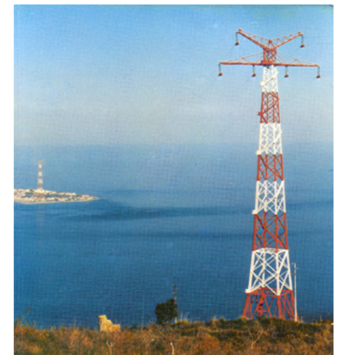
The electric crossing of the Strait of Messina, built in 1955 and put out of service in 1994.
