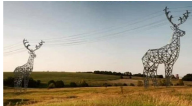
Transmission line with zoomorphic supports.
