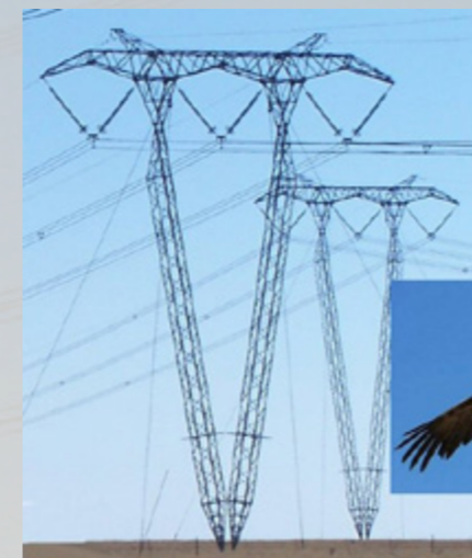
Supports of 765 kV lines in South Africa, with eagle wing cross arms.
