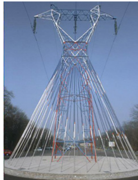
Dressing of a 220 kV line pylon near the spa town of Amnéville les Thermes, in the north of France, designed by Elena Paroucheva.
