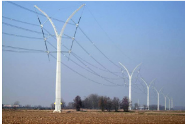
Support Dutton-Rosental (bud pole) for a 380 kV transmission line in Italy.
