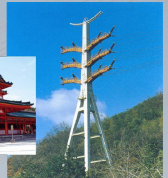
Support with curved cross arms like the traditional roofs of oriental buildings.
